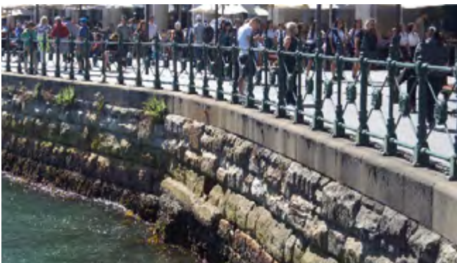
Circular Quay seawall. Source: L Chaffer
