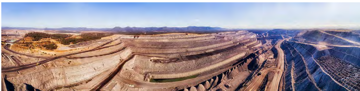
Elevated aerial panorama over deep excavation at an open cut coal mine in the Hunter Valley. Source: Shutterstock
