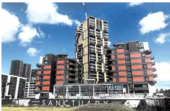
Sanctuary Apartments, Wentworth Point
